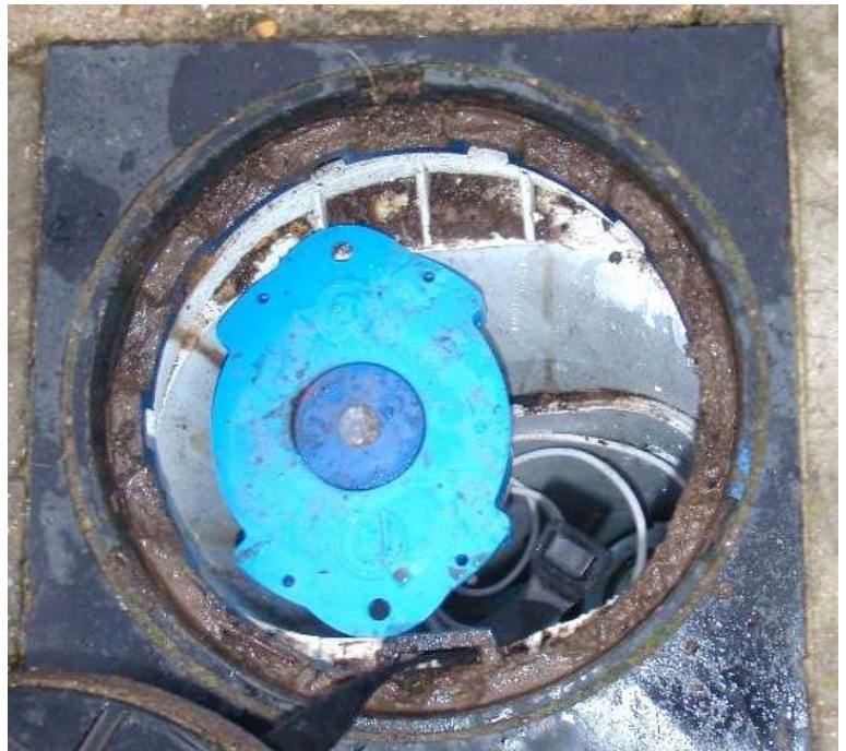
Figure 14. Logger in Talbot round lid box example
