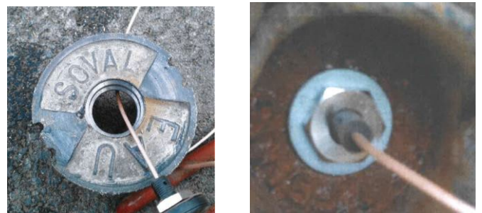
Figure 31. Thread antenna into position and secure in place with supplied nut and a suitable washer
