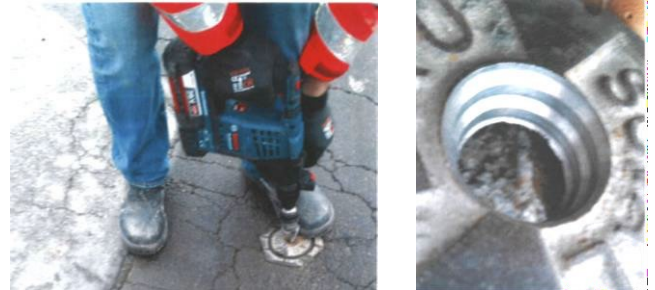
Figure 30. Drill hole and recess in chamber lid
