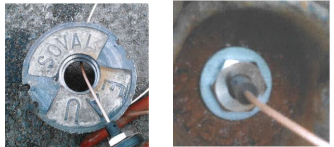
Figure 20. Thread antenna into position and secure in place with supplied nut and a suitable washer
