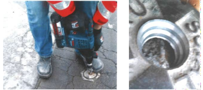
Figure 19. Drill hole and recess in chamber lid
