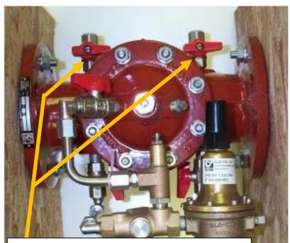
Stop Taps (for service): Close those required for transducers and water feed to Hydroswitch solenoid valve.
