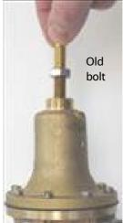
Unscrew and remove the existing PRV pilot adjustment bolt. (see picture). Check the outlet pressure reading whilst removing the bolt; the pressure should not change. If pressure drops at this point a valve is leaking.
