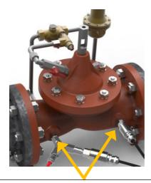
Open service valve that provides Hydroswitch water feed and any that connect to external transducers.
