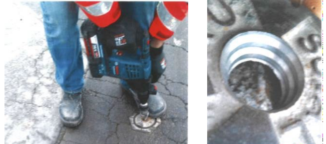
Figure 30. Drill hole and recess in chamber lid
